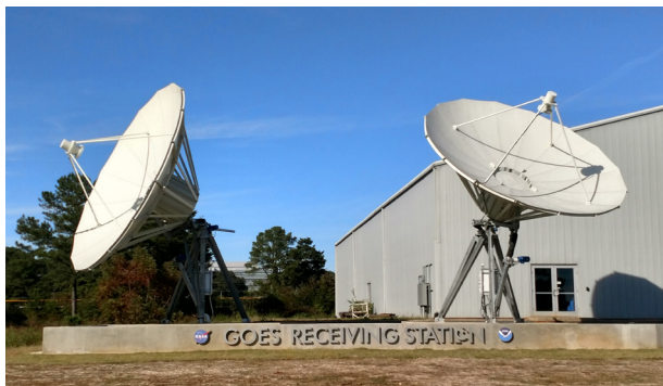
GOES Receiving Station at Marshall Space Flight Center, Building 4316.
